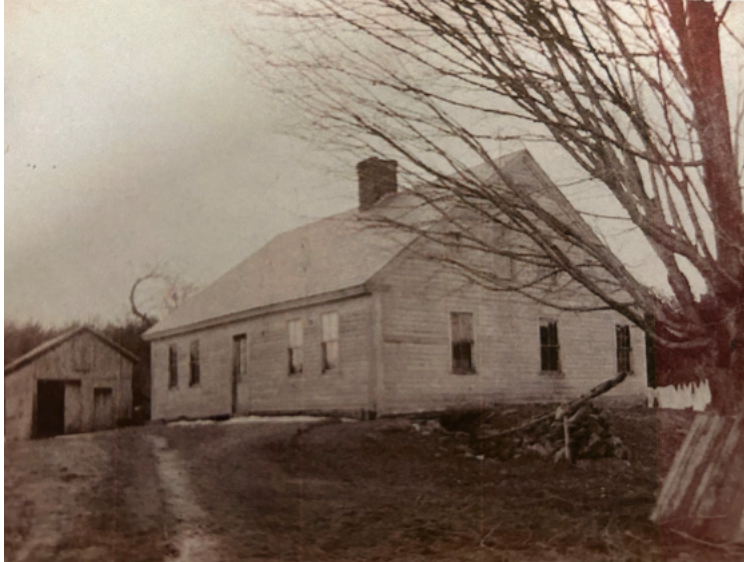
Early picture of 1204 Buckley Highway
